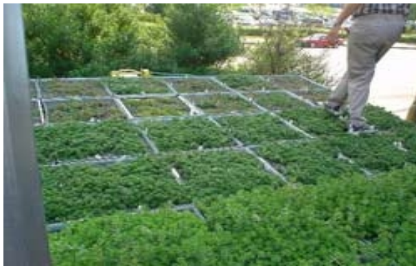
Green Roof Blocks system with modular 2 x 2 aluminum planters.
