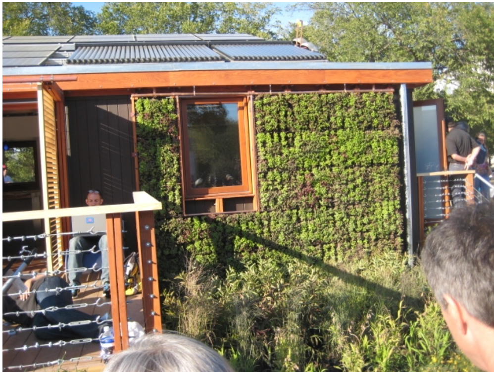
“Vertical rain garden” or green wall on University of Maryland demo home entry in the DOE Solar Decathlon, 2007. Photo: Alarcón
