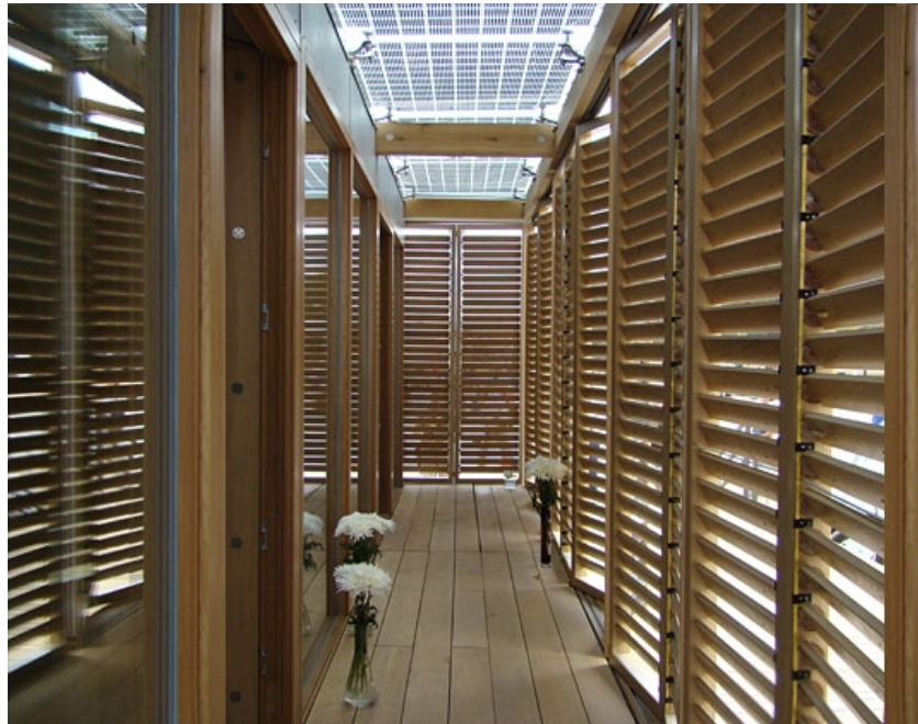
Solar shutters on Darmstadt University entry. Source: Inhabitat.com
