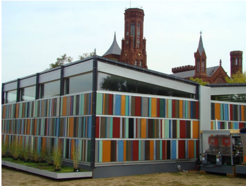
Rain shell made of salvaged steel roofing from University of Cincinnati. Source: Inhabitat.com
