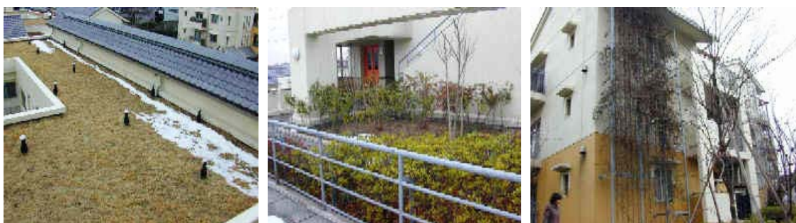
Green rooftops and walls
