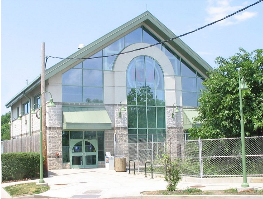
Figure 1: The new W. 65 th Street RTA station
