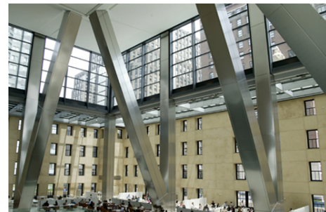
Old & New Structure – from inside
