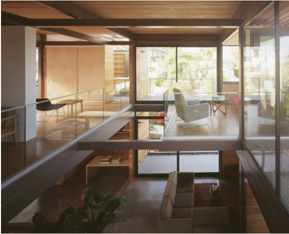
The window glass contains low-e glazing to help keep heat out in the summer and retain it in the colder months. (Source: www.livinghomes.us )
