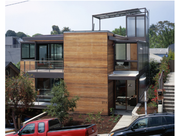
The rooftop solar pannels generate energy for the home. (Source: www.livinghomes.us )
