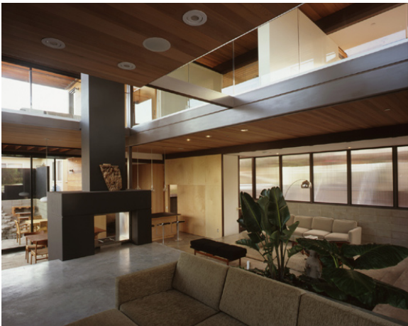
The structure of the house is made from steel, which is not susceptible to mold like stick frames are. (Source: www.livinghomes.us )
