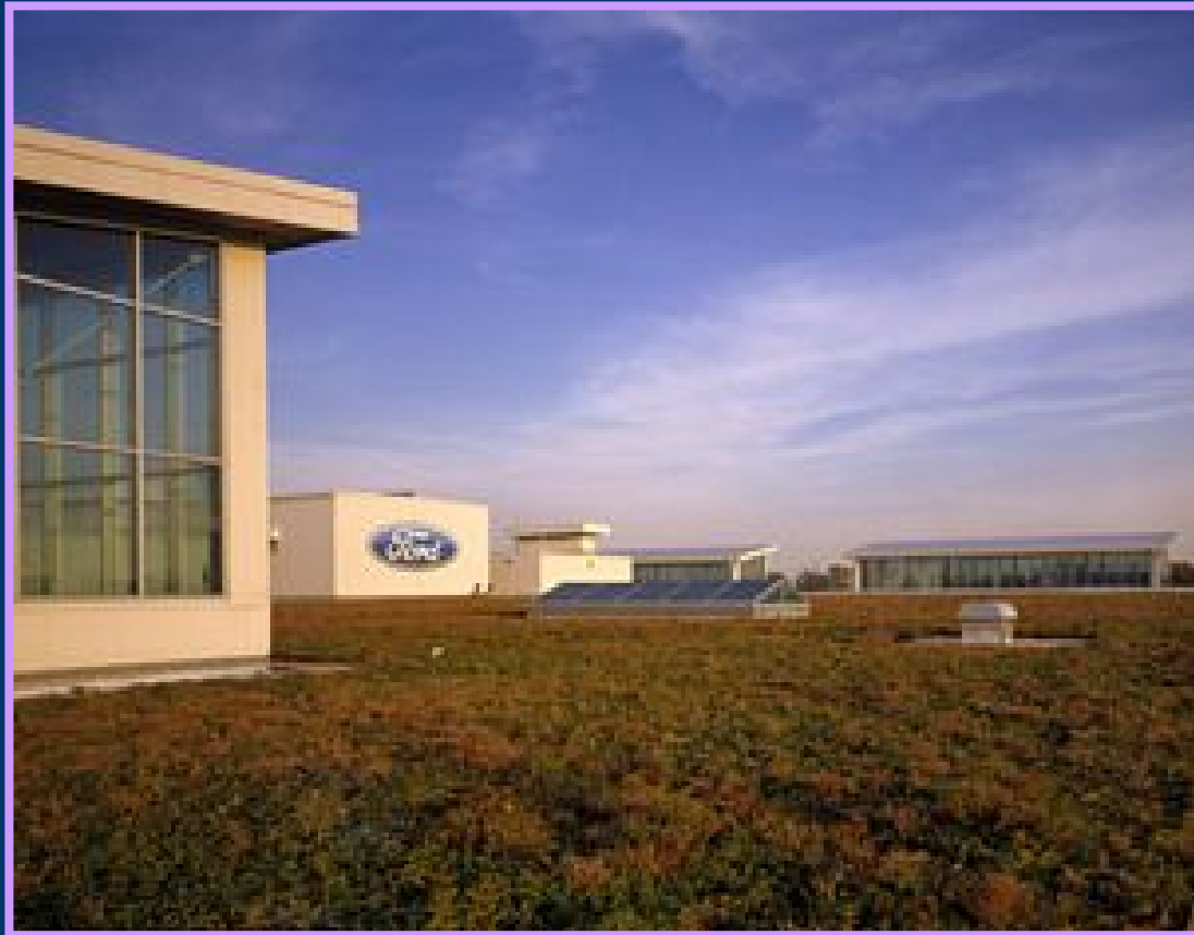
Ford Rouge Plant's day-lighting window boxes that look out to the green roof
