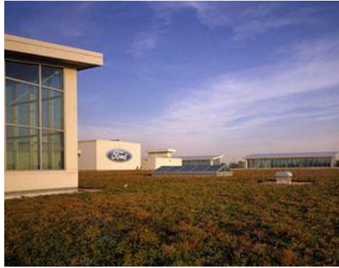
Figure 5. Daylighting window boxes that look out onto the living roof (AIA Michigan).
