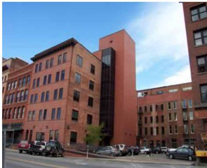
Figure 1 The Alliance Center sits near 15 th and Wynkoop Streets in Denver, Colorado
