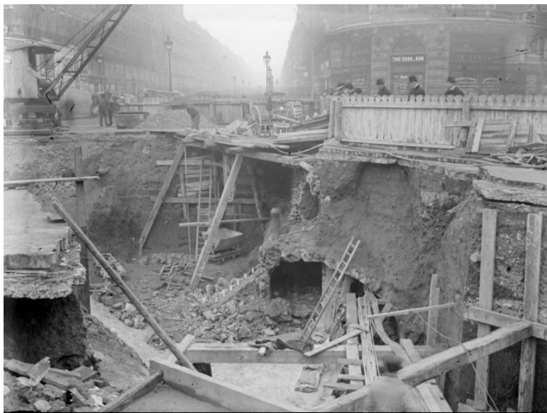
Constructing the Métro involved tearing up many streets (7).
