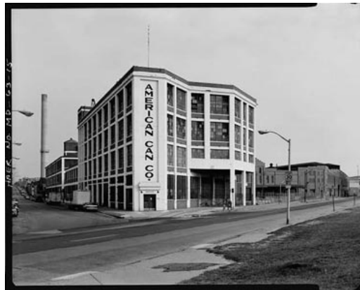
Figure 1: The original Can Company's flagship building. ( thecancompany.com )
