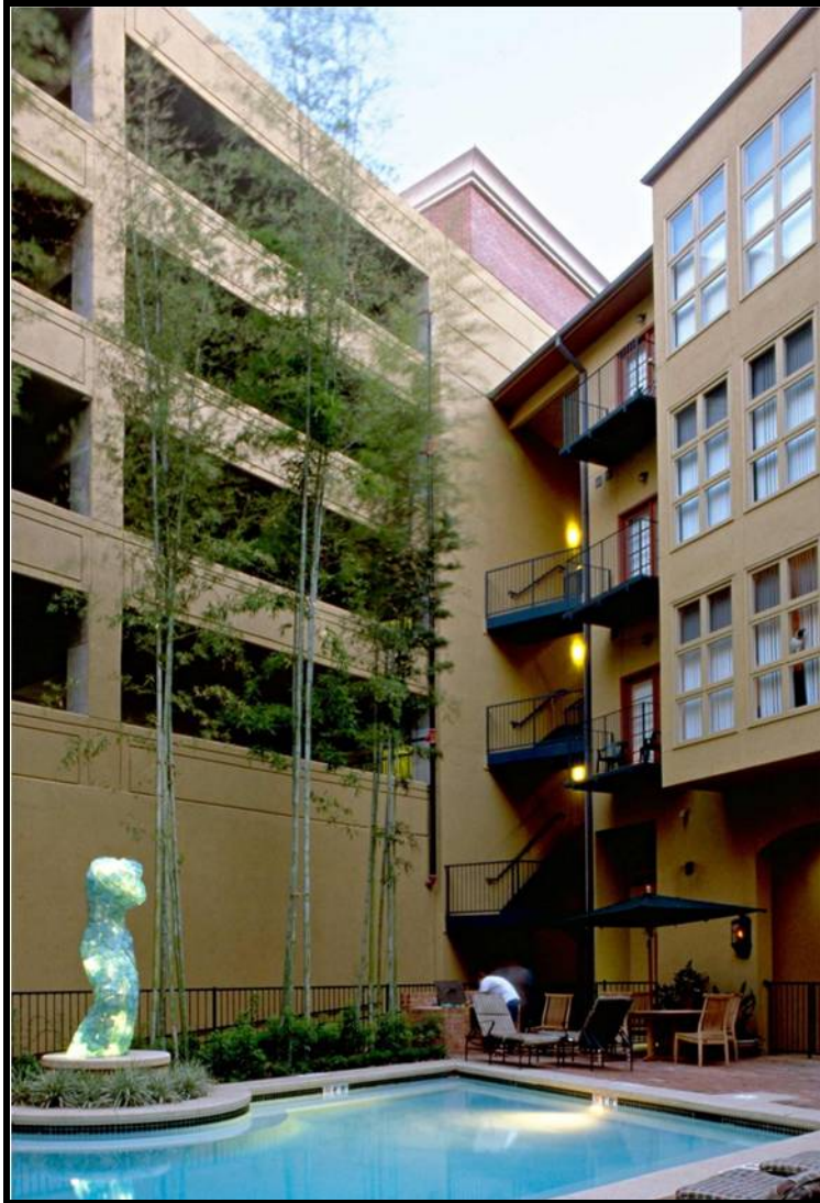
Figure 7. Parking Structure at Addison Circle, Source: David Whitcomb/RTKL
