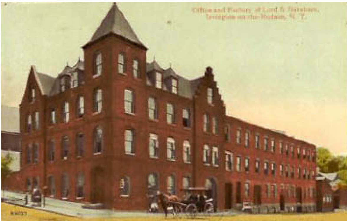
Burnham Building – Early 1900's
