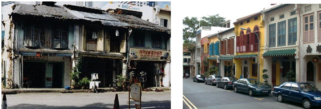
Figure 4. Dilapidated, crumbling shop-houses in Chinatown (left) and cleaned, restored shop-houses post-redevelopment (right). (George P. Landow, G.P. and Rosenthal, J.C.)
