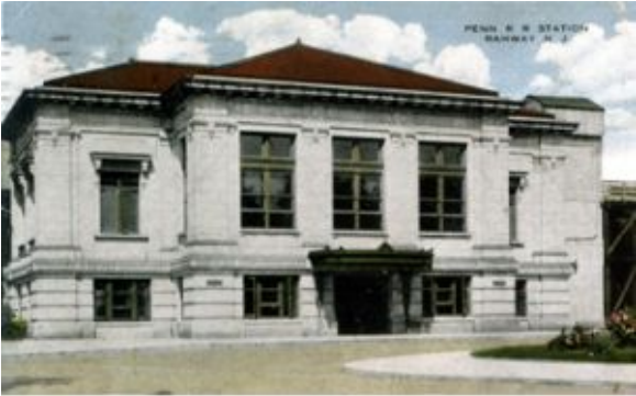
PRR Station, 1920s
