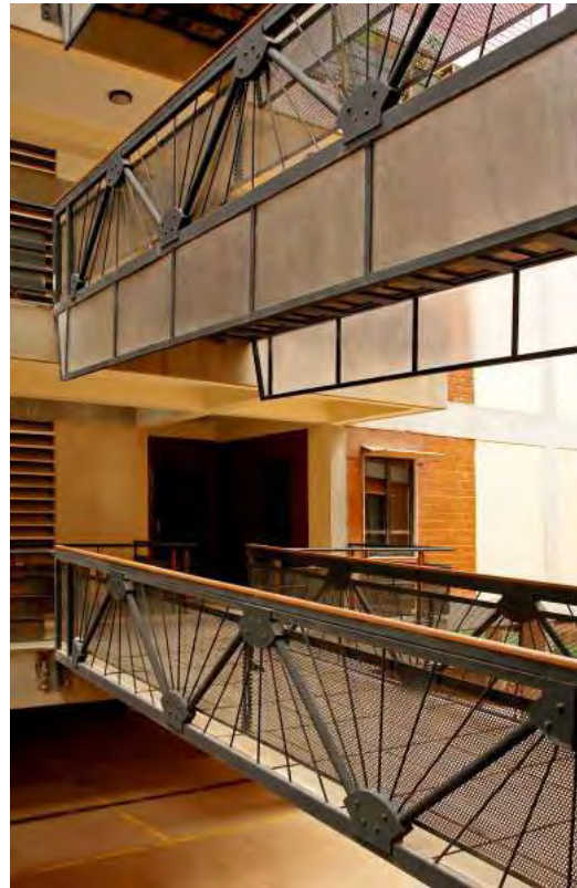
Fig 7 Steel staircase connecting apartments
