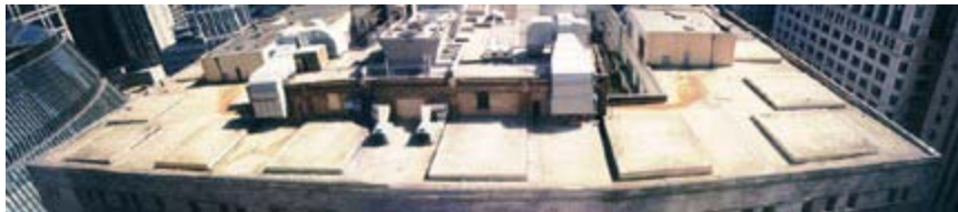
City Hall "Before"
