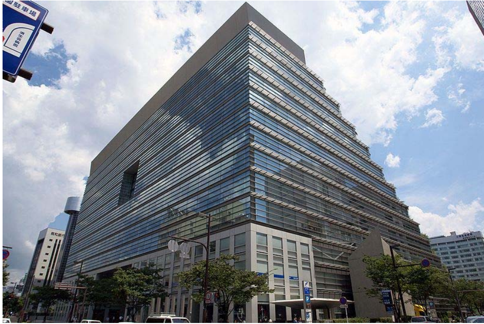
North side: modern office building
