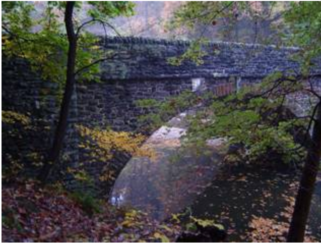
Bridge over Wissahickon Creek, Hecker
