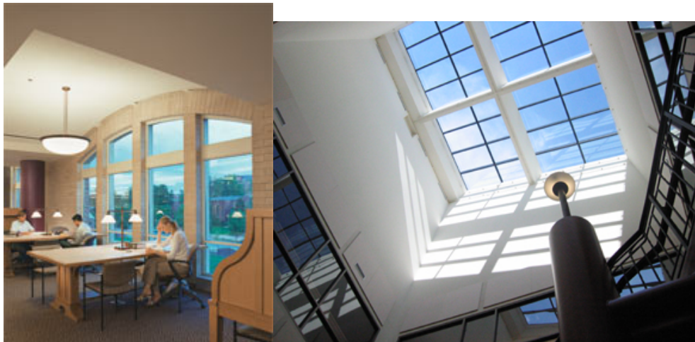
Light harvesting: large windows on walls and the ceiling allow ample natural light into the building, thereby reducing the need for electric lighting. Source: H + Architecture ( www.hlarch.com )
