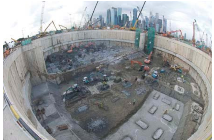
Pile caps under construction within the Tower One.
