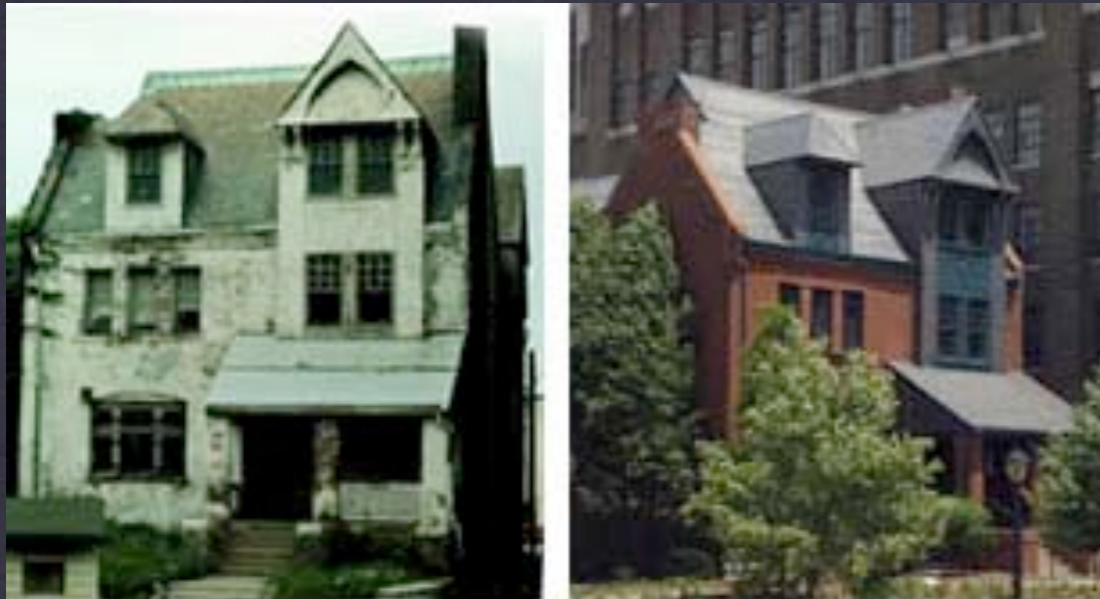
Renovation Raw Material The EarthWays Home "Before" and "After"
