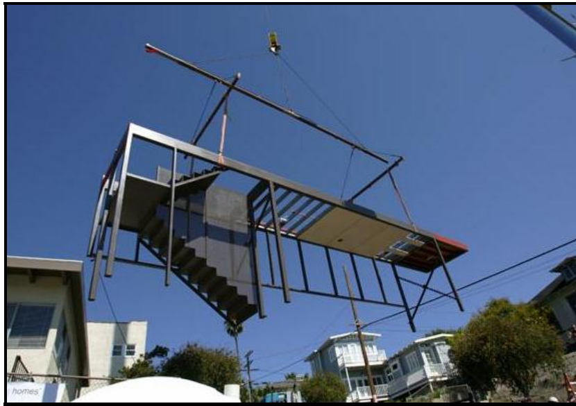
Figure 6. On-Site Assembly of Prefabricated Components. Source: www.livinghomes.net
