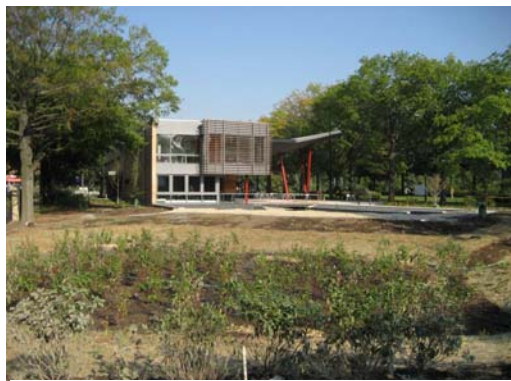
Bioswale on western side of building. Photo from QBG website
