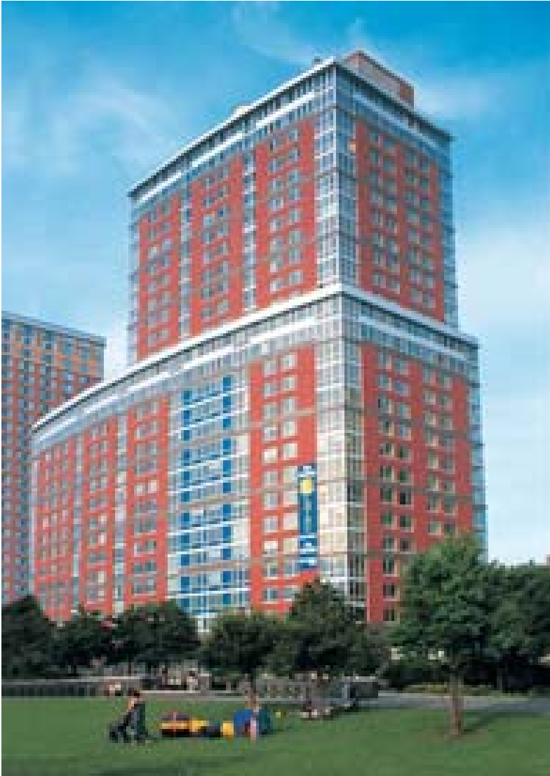
A front view of The Solaire. The characteristic blue panels on the front are the photovoltaic cells. ( http://www.batteryparkcity.org/ )
