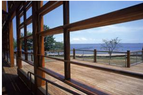
Figure 3: External louvre system made from recycled pickle barrels (Griffith et al 2005).
