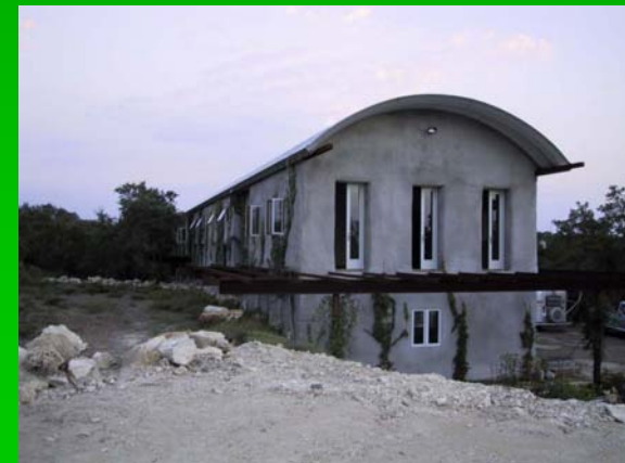
Villa Millenium, Bee Creek Texas Under Construction 2001
